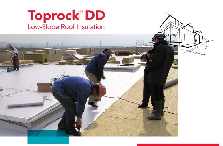
ROCKWOOL Toprock® DD is a rigid and high-density, uncoated stone wool insulation board for low-slope roof applications. Toprock DD is a suitable substrate for mechanically-attached membrane systems in low slope roofing.
