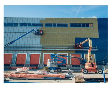
When exposed to clement weather conditions, ROCKWOOL unfaced exterior wall insulation products, when installed vertically, may remain exposed for up to 90 days without negatively affecting their properties. Faced insulation product Cavityrock® Black, may be exposed for up to 30 days without adverse effects.
