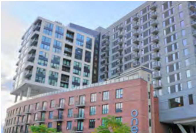
Panelized EIFS One Seven at Bellevue Station Denver, Colorado
