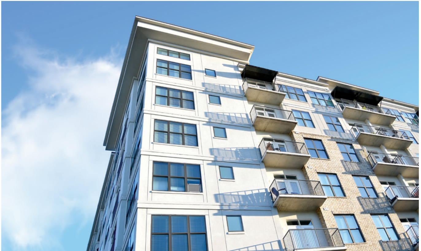
Senergy Wall Systems can create a multiple cladding appearance with continuous exterior insulation and a seamless air/water-resistive barrier
