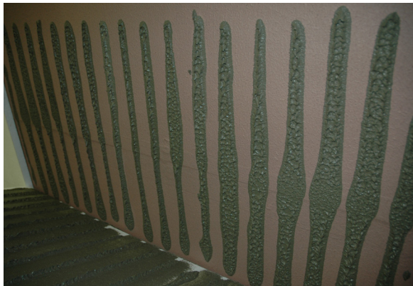
Typical example of troweled adhesive transferred to the substrate, creating channels for drainage.
