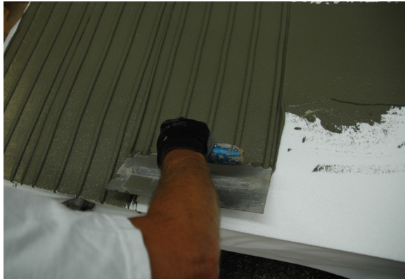
Cementitious adhesive/base coat properly applied in vertical ribbons to back of EPS board.
