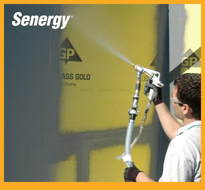
Framed Construction Incorporating Fluid-Applied Senergy Air/Water-Resistive Barriers
