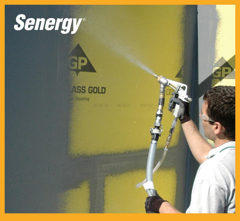
Framed Construction Incorporating Fluid-Applied Senergy Air/Water-Resistive Barriers Typical Details
