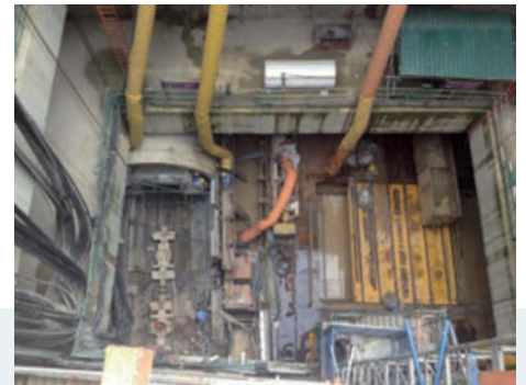
Figure 25 : DTL3 C933 – East TBM launch shaft at Bendemeer station
