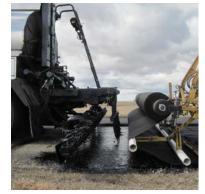
Propex pioneered paving interlayer fabrics with **PETROMAT Original** fifty years ago. Today it continues to be the most proven asphalt paving fabric in the market. No other product provides a better pavement moisture barrier or stress absorbing interlayer to prevent reflective cracking.
