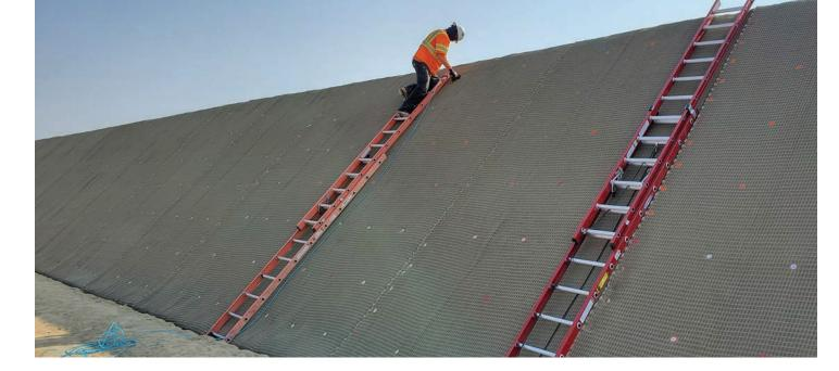
PYRAMAT® 75 High Performance Turf Reinforcement Mat and PYRAMAT® 25 Turf Reinforcement Mat are erosion control solutions engineered to mitigate the risk and increase resilience of wildfireprone areas through non-halogen fire retardant technology.
