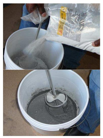
While mixing for 3 minutes stop to scrape down the sides to insure all material is fully mixed
