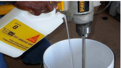
Mix liquid thoroughly for 30 seconds with a Sika paddle (jiffy mixer) on a low speed drill 400-600 rpm drill.
