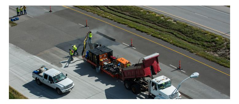
High Friction Surface Treatment (HFST) is a single layer epoxy application with high friction aggregate that significantly and immediately increases roadway friction to reduce auto crashes, injuries and fatalities on problem road surfaces.
