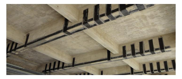
SikaWrap and CarboDur composite materials are constantly used in critical applications to solve challenging structural problems, including but not limited to confinement and shear strengthening, seismic upgrades, impact and blast resistance, and design or construction defects.
