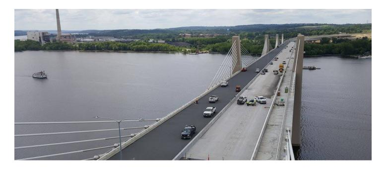
Thin Polymer Overlays (TPO) provide a high-friction, long-lasting wearing course on concrete bridge surfaces that protects the deck from moisture and deicing salt penetration, inhibiting future corrosion.
