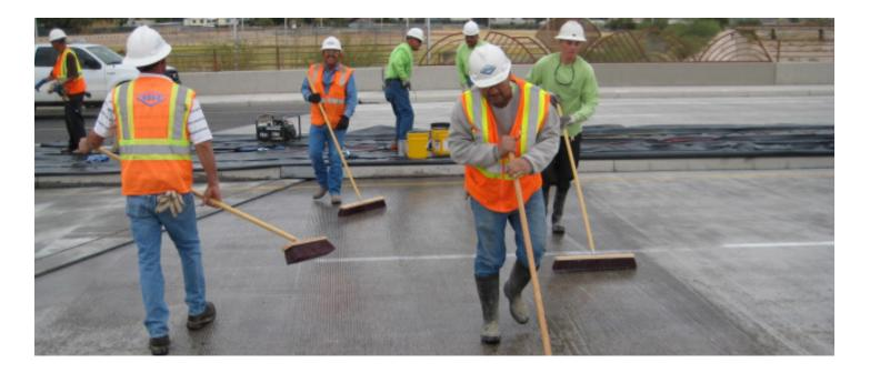
Epoxy crack repair applications are structural and economical solutions for cracked and unsound concrete that will prolong the life cycle of any existing structure. These can be used alone or in conjunction with other repair and protection systems.
