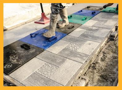
**STAMPED OR COLOR HARDENED CONCRETE:** Spray apply uniformly onto the concrete surface in two equal applications as follows:
