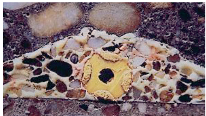
Joint waterproofed and sealed
