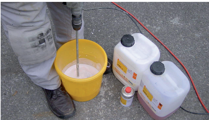
Mixing of an acrylate injection resin
