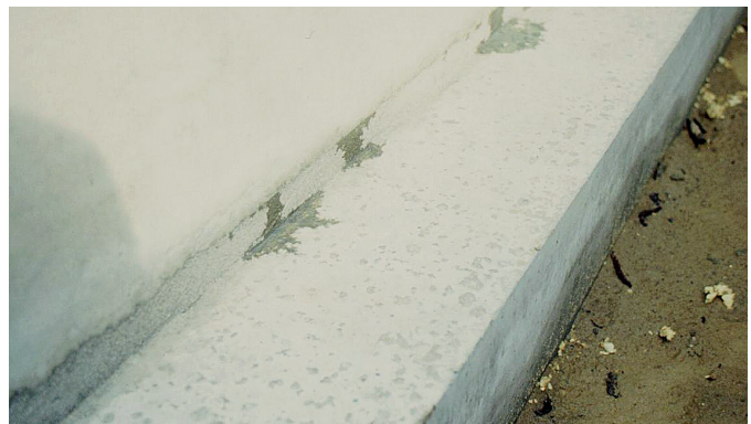
Simple injection process on site
