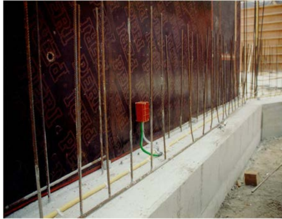
Figure 2: vent ends entering junction box
