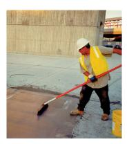
3. The longer working time of SikaQuick 1000 makes this product more conducive to larger areas of placement. Final broom finish provides for a slightly roughened surface and skid-resistance that is desirable on parking decks.
