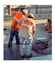
2. SikaOuick 1000 poured into place and mechanically screeded.
