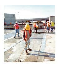
1. Scrub coat of SikaOuick 1000 is completed just prior to the placement of the overlay. This step is always required in concrete repair to ensure excellent adhesion to the existing substrate.
