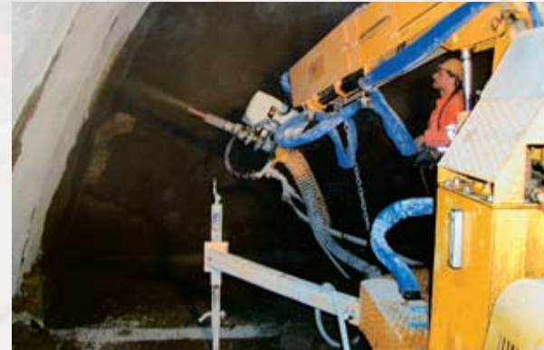
Aliva-503 shotcreting system for small sections
