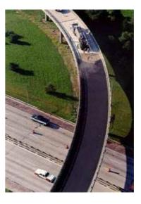
– U.S. 40/I–64, a doubledeck bridge complex in downtown St. Louis and critical east—west link across the Mississippi River, recently had its existing asphalt overlay removed and replaced with a Sikadur 22 Lo–Mod polymer concrete overlay. This project is the largest of its kind completed anywhere in the world.
