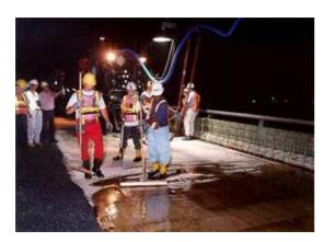
The Sikadur polymer concrete overlay also provided rapid turnaround, which allowed the contractor to install the overlay at night and then reopen the roadway.
