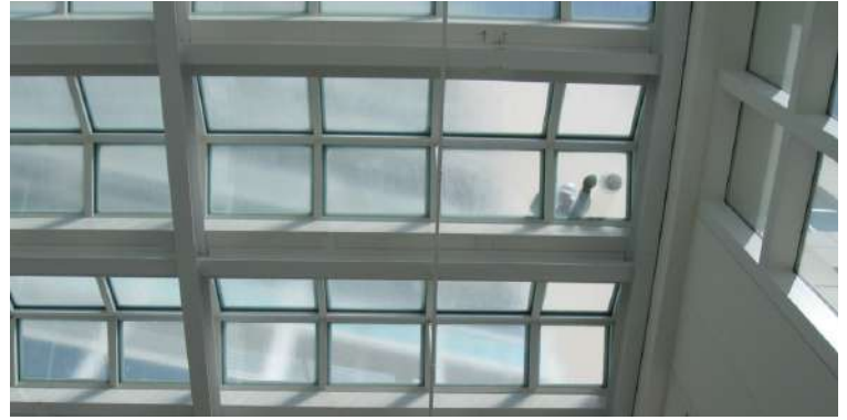
Appearance of clearglaze applied to existing skylights.
