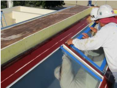
Remask the picture frame and apply Sikalastic® RoofPro resin to the primed surface of the mullion and glass.
