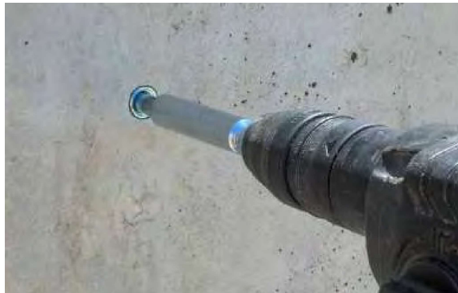
Anchor being set with SDS setting tool.
