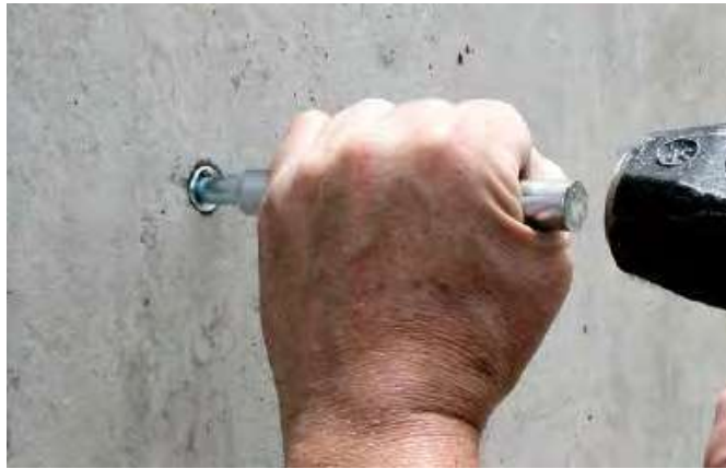
Anchor being set with hand setting tool.
