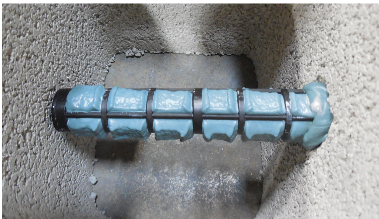
Hollow CMU Install with Opti-Mesh Screen
