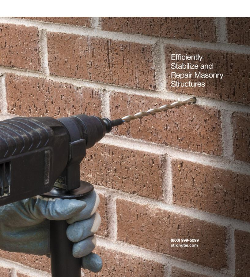
The Heli-Tie helical wall tie is a stainless-steel helical tie used to anchor building façades to structural members or to stabilize multiple-wythe brick walls.
