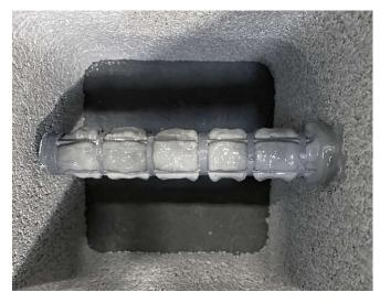
Specially sized holes in Opti-Mesh screens allow for adhesive to seep out at the appropriate location at the hollow portion of the CMU to create a better bond to the face shell.
