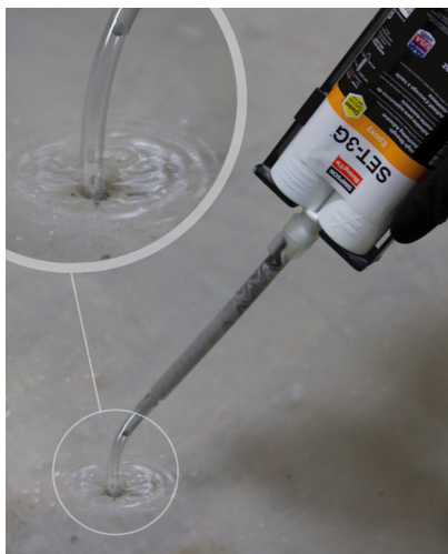
Submerged concrete hole installation.
