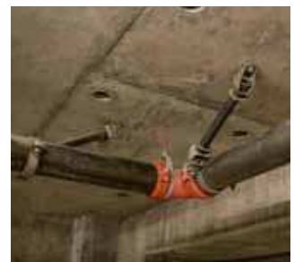
Seismic Bracing
