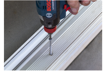
Sliding door track installation
