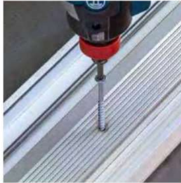
Sliding door track installation
