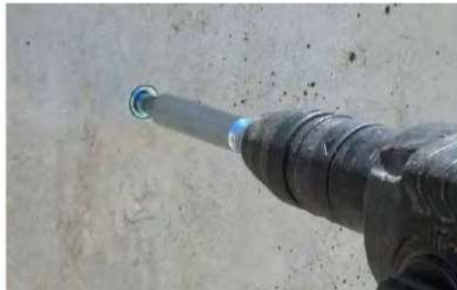
Anchor being set with SDS setting tool.
