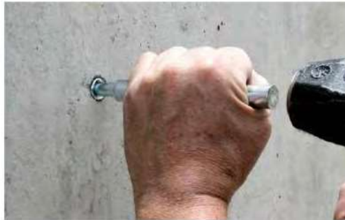
Anchor being set with hand setting tool.
