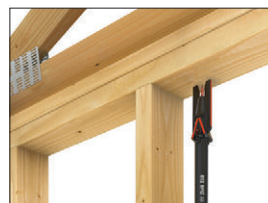
Gable end truss installation.
