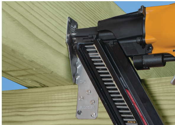
Strong-Drive 33° SCNR Ring-Shank Connector Nail (paper collated)
