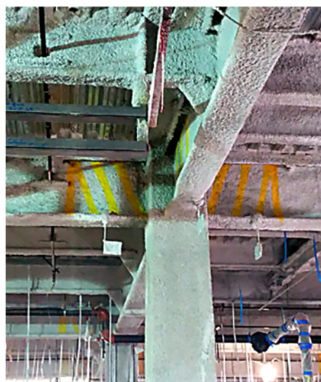
Figure D4b.3 — Protected Zone Marking for an RBS Connection in the Field (Sprayed on Top of Fireproofing)
