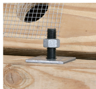
Separation Between Nut and Bearing Plate Due to Wood Shrinkage
