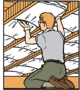
Typical IS Installation
