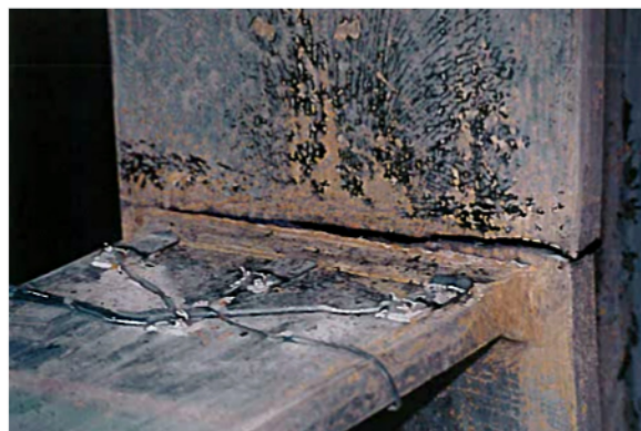
Figure D2.3 — Fracture of Welded Beam-to-Column Connection in a Laboratory Test
