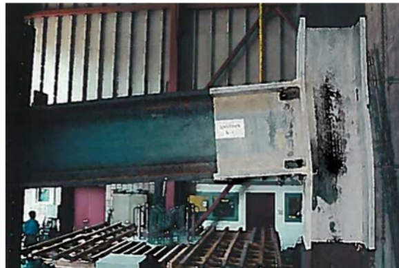
Figure D2.1 — Column Kinking Attributable to Weak Panel Zone
