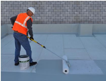
4. Embed a layer of Pro Fleece into the base layer of wet Paraflex Liquid Membrane.
