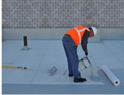
2. Apply a base coat of Paraflex Liquid Membrane using an approved roller or stub roller. Refer to the chart on page 11 for application rates.
