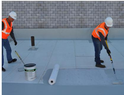
5. Use a roller to fully embed the fleece into the liquid membrane and remove trapped air. Lap fleece layers a minimum of 2 inches, and apply an additional coat of Paraflex Liquid Membrane between layers of overlapping fleece.
