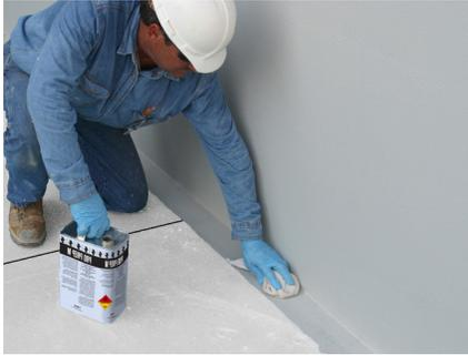
1. Using Pro Prep M, wipe/clean existing Paraflex surfaces to receive an overlap of the Paraflex materials. Allow Pro Prep M a minimum 20 minutes drying time after application before continuing.
