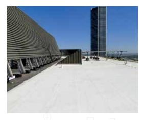
Bright white, liquid-applied Parapro PMMA Roof Membrane offers cool roof benefits with exceptional durability.
