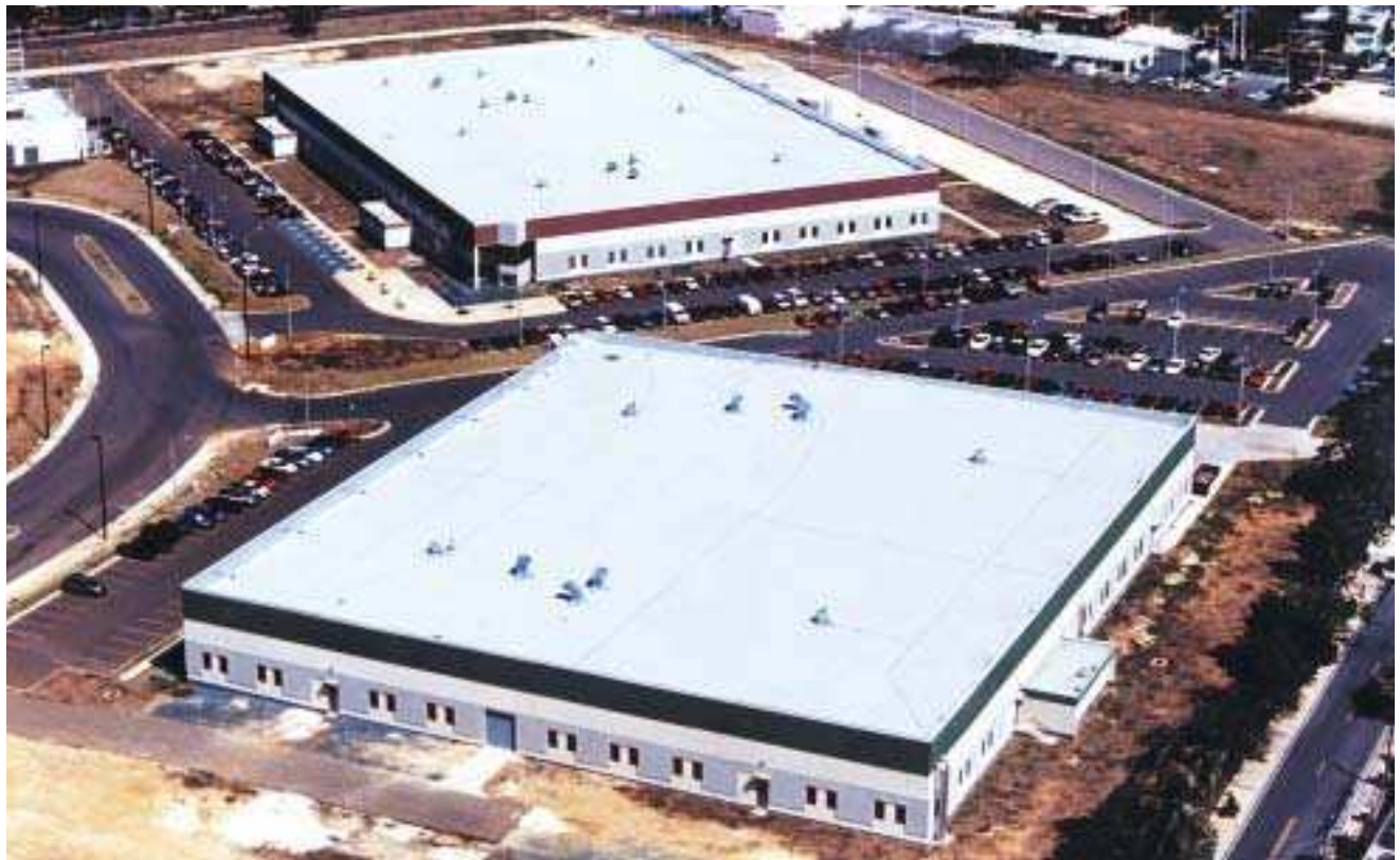
Over 700 squares of Paradiene were applied in PA-311 Adhesive on this office facility in Puerto Rico.
