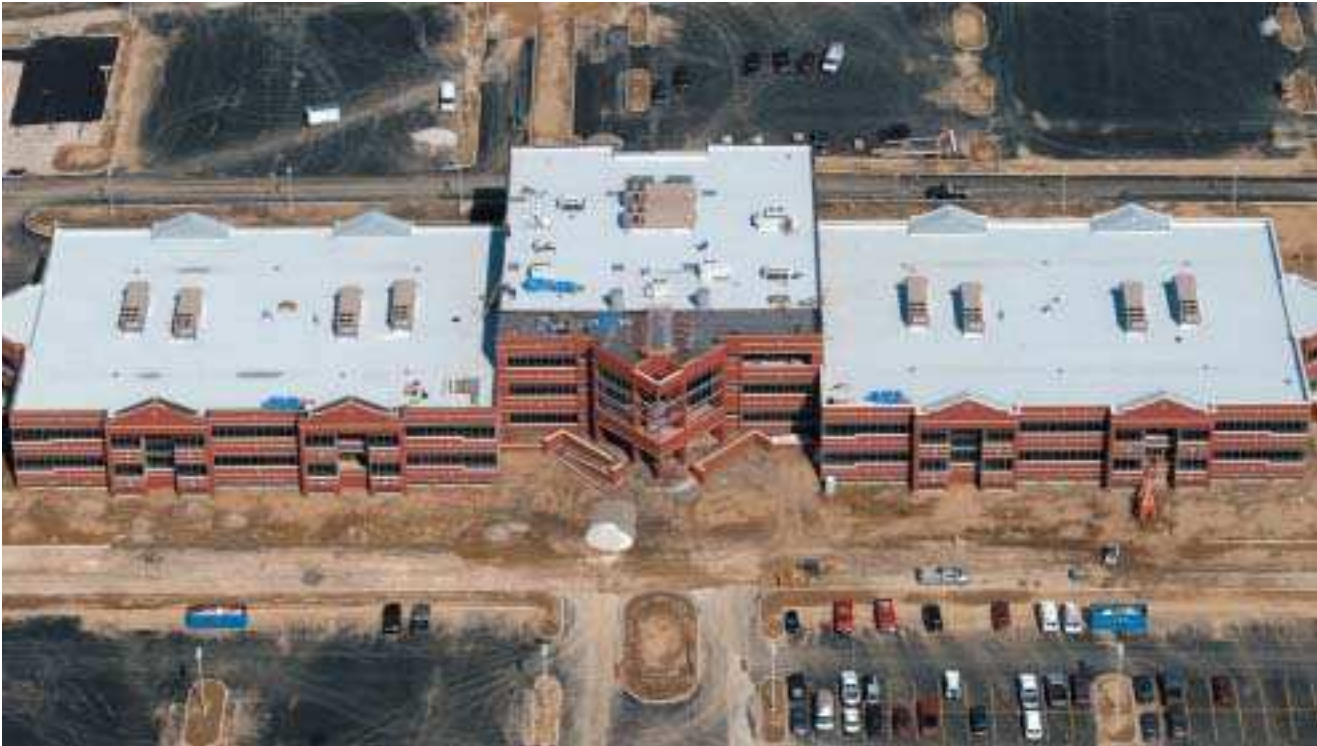
A Paradiene 20/30 system was applied in PA-311 Adhesive on this Ohio facility.
