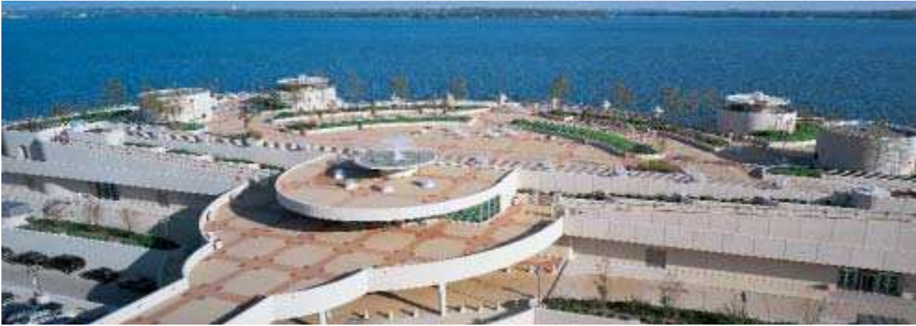
The Teranap Waterproofing System was chosen for the plaza deck of Frank Lloyd Wright's Monona Terrace in Madison, Wisconsin.
