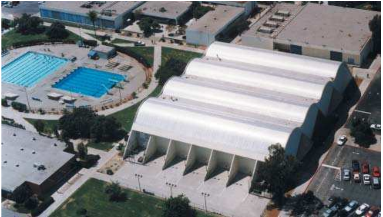
Energy efficient, aluminum foil-faced Veral was used to create the reflective roof on this facility on the campus of a California college.
