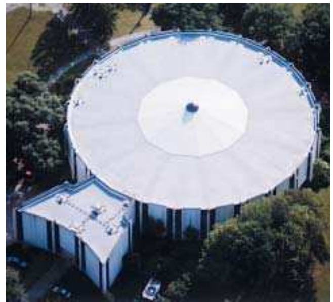
A Paradiene 30 TG/ 30 FR TG system and energy efficient Polar White Veral Spectra protect the collection of this library on the campus of a Georgia university.
