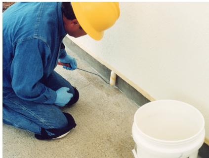
1. Using tape, mask the perimeter of the area to be flashed to ensure a clean edge. Prime the substrate with Pro Primer (type depending on substrate) and allow to cure for 45 minutes.
