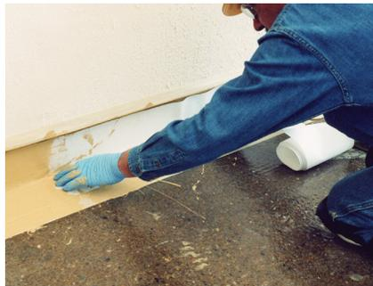
2. Over the primed substrate, apply a base coat of catalyzed Terapro Flashing Resin with a roller or brush. Work Pro Fleece reinforcement into the wet, catalyzed flashing resin base coat using a roller or brush to fully embed the fleece in the resin and remove trapped air.
