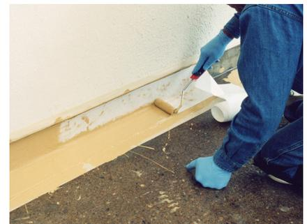
3. Apply an even top coat of Terapro Flashing Resin immediately following embedment of the fleece to ensure full saturation of the fleece. Remove tape before the resin sets.
