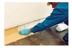
Over the primed substrate, apply a base coat of catalyzed Terapro Flashing Resin at a minimum rate of 0.19 kg/sf - 18.6 kg/sq (2.0 g/m²) with a roller or brush. Work Pro Fleece reinforcement into the wet, catalyzed flashing resin base coat using a roller or brush to fully embed the fleece in the resin and remove trapped air.
