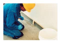
Using tape, mask the perimeter of the area to be flashed to ensure a clean edge. Prime the substrate with Pro Primer W or Pro Primer T (depending on substrate) at a minimum rate of 0.037 kg/sf - 3.7 kg/sq (0.4 kg/m²). Allow to cure for 45 minutes.
