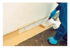
Apply an even top coat of Terapro Flashing Resin immediately following embedment of the fleece at a minimum rate of 0.12 kg/sf - 12.1 kg/sq (1.3 kg/m²) to ensure full saturation of the fleece. Remove tape before the resin sets.
