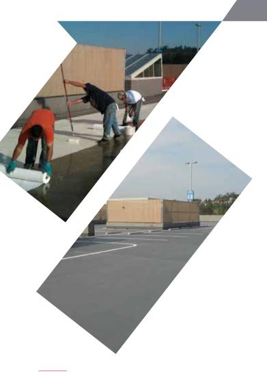
The Terapro VTS system provides a high performance solution to the demanding waterproofing challenges of parking deck applications like this one, on a large shopping mall in the Pacific Northwest.
