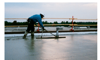
Siplast Lightweight Insulating Concrete is screeded to a smooth, durable, monolithic surface ideal for roofing application.
