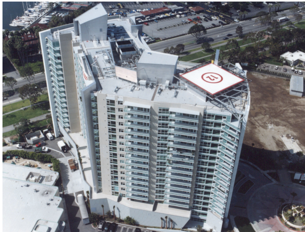
This high-rise luxury condominium tower on the beach at Marina Del Rey, California is protected by a complete Siplast System of torch grade Paradiene and Siplast Lightweight Insulating Concrete.
