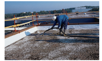
On this reroofing project, a thin slurry coat of lightweight insulating concrete is poured in place, correcting substrate irregularities and bonding the Insulperm Insulation Board to the substrate.
