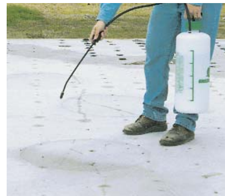
Moisten the existing substrate with water.
