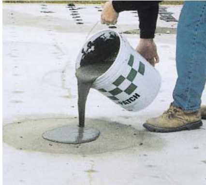
For thin patch repair, pour Zono-Patch into place.
