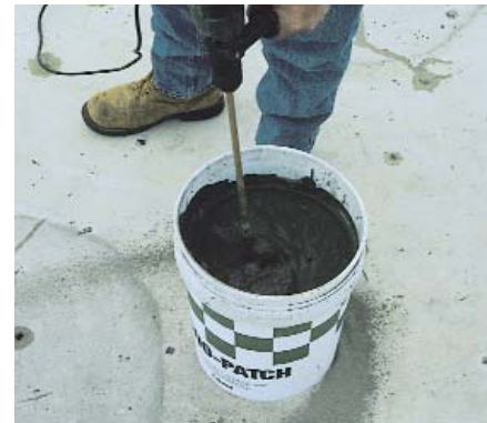
Using a mortar mixer or "jiffy" mixer, mix to a smooth, creamy consistency.
