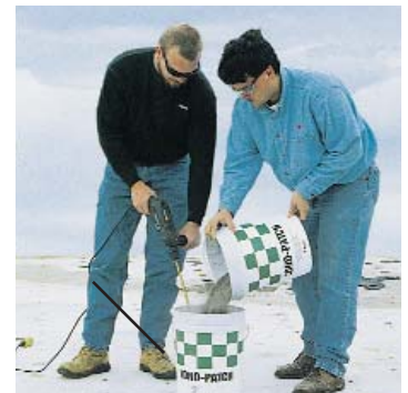
When mixing Zono-Patch, always add dry powder to water.
