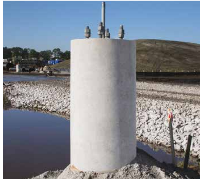
Sonotube Finish Free form column
