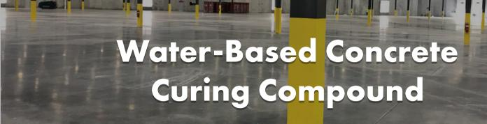
E-Cure<sup>®</sup> is a leading edge technology, clear concrete curing compound that was developed to cure concrete as well as resolve compatibility issues related to flooring adhesives. E-Cure<sup>®</sup> is a spray applied concrete cure, hardener and dustproofer.
