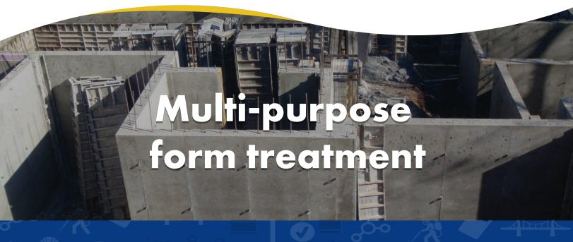
EZ CLEAN & RELEASE is a ready to use highly reactive petroleum mixture that, when properly applied to concrete forms with concrete build-up, will soften the hardened concrete and "self-clean" as the forms are stripped.
