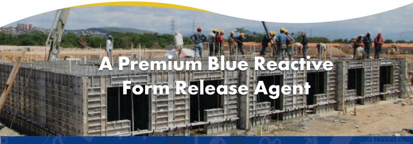
A chemically active concrete form release agent specifically designed for use on aluminum forms. The reactivity of Ultra Blue is perfectly matched to do the challenging job of ensuring a clean release on pour while keeping aluminum forms free of concrete buildup. Protect and maximize the utility of your aluminum forming investment with Ultra Blue.
