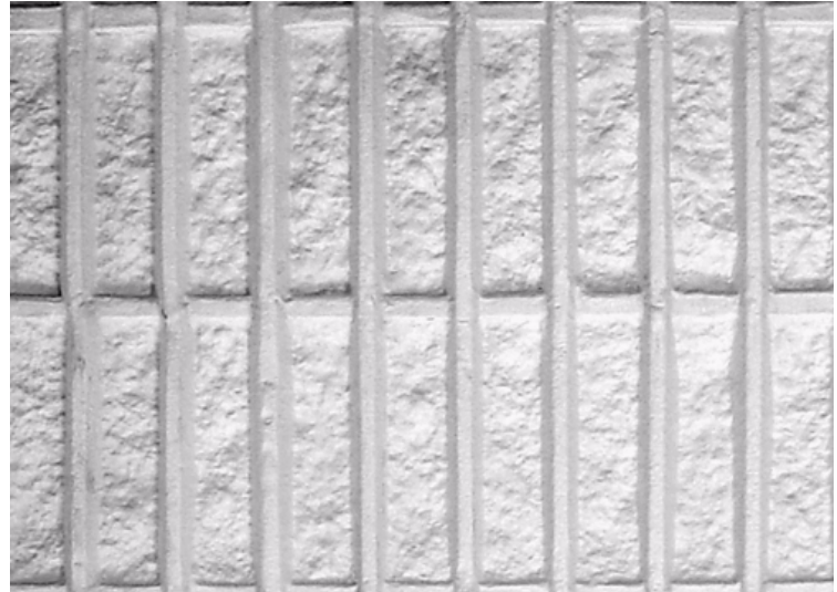
8" x 16" split rib block - ribs average depth 3/4" - mortar joint average 1/2" depth. 4' x 8' panels.
