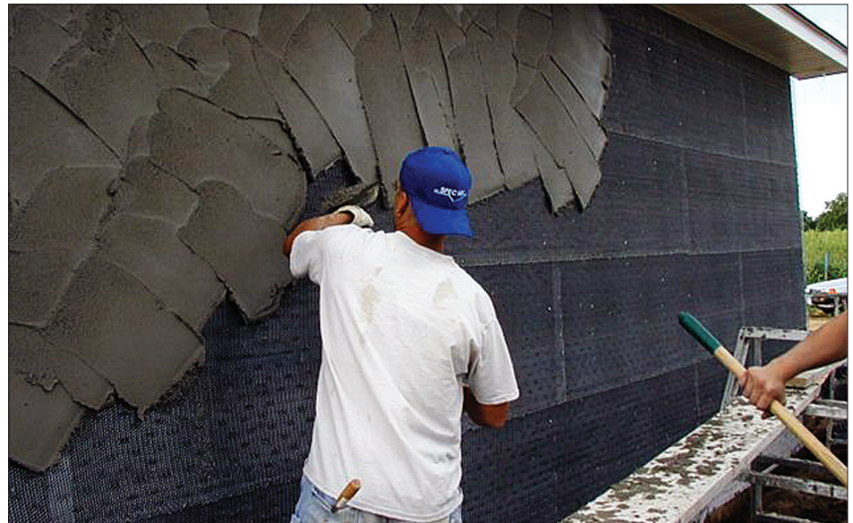
Application of proprietary, preblended, shrinkage compensated basecoat
