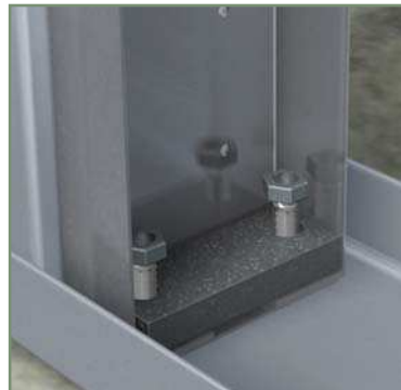
Install nuts/washers on anchors.
