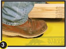
Apply downward pressure for 5 to 10 seconds; Beast Foot's engineered adhesive is pressure sensitive. (Tip: In cold weather, extra time may be needed while applying pressure).
