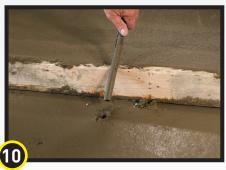
Beast Form Stakes can be removed once concrete has set sufficiently to hold its own shape. (Beast Form Stakes are designed to be reusable).
