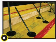
Spacing to be determined by the contractor depending on the depth of the concrete. (Follow standard construction practices; however, spacing should not exceed 3' to 4').
