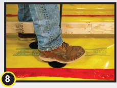
Remove the Pull Tab and apply Beast Foot to the vapor barrier, remembering to apply downward pressure.
