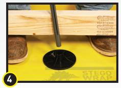
Install Beast Form Stake into the press-fit center hub of Beast Foot; be mindful of the positioning of the fastening grooves.
