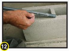
Once concrete has dried on Beast Form Stake, strike it against a hard surface to loosen the concrete buildup. Rub off the remaining concrete with a glove or dry rag. The fastening grooves should be kept free from excess concrete buildup.
