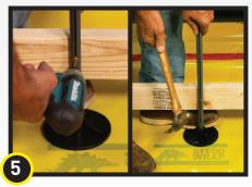
Fasten the Beast Form Stake to the form with a duplex nail or self-tapping screw. (Use up to 8D duplex or up to #8 screw).
