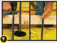
Secure form in position using a nail or screw. (The 18" length of Beast Form Stake will allow a maximum form height of 12" to top of form – above the vapor barrier).
