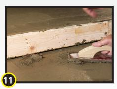
Fill and repair any voids in the concrete as necessary once the Beast Form Stakes have been removed.
