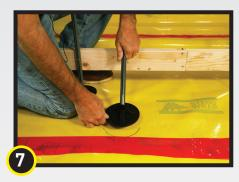
For lateral bracing, position Beast Foot so a 45-degree angle is established between the form and Beast Form Stake. Beast Form Stake threads onto the "Side Boss" of Beast Foot for form bracing. (Tip: Attach Beast Form Stake and mark position prior to removing Pull Tab).
