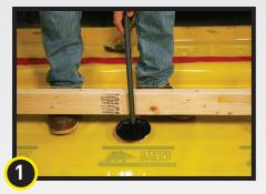
Ensure the press-fit center hub of Beast Foot is positioned in line with the form to be set. (Tip: pulling a string line or snapping a chalk line can be a helpful aid).
