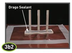
Pour Drago Sealant inside of Drago Sealant Form to create a seal around the penetrations.
