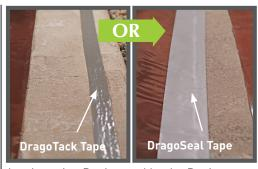
At a Location Designated by the Design Team: Seal Drago Wrap to concrete with **DragoTack Tape or DragoSeal Tape**.
