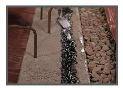
Onto Interior Grade Beams at Impediments: Seal Drago Wrap to concrete with Drago Mastic.
