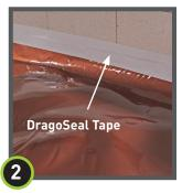
Apply **DragoSeal Tape** on the perimeter edge so that 2" is on the Drago Wrap and 2" is on the wall/vertical surface. Press firmly to secure.
