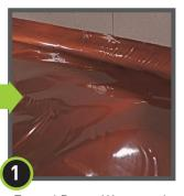
Extend Drago Wrap up the vertical surface, likely to the height of the slab.
