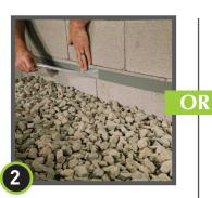
When ready to apply Drago Wrap, remove the exposed release liner from **DragoTack Tape**.
