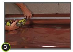
Fasten a termination bar over the top of the Drago Wrap inline with the Drago Mastic.
