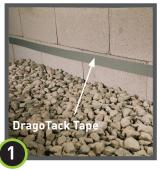
Remove the release liner on one side of **DragoTack Tape** and adhere to foundation wall at the height of the slab or at impediments.
