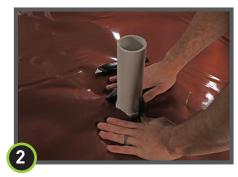
Pull material over and flatten. Clean area of adhesion where the Drago accessory will be applied.
