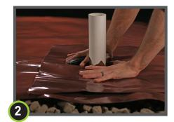
Cut an "X" the size of the pipe diameter in the center of the detail patch and slide tightly over pipe.
