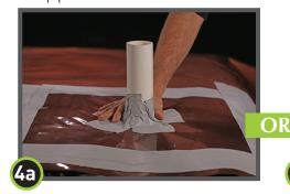
Seal around the base of the pipe using DragoSeal Tape.
