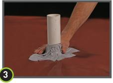
If Drago Wrap is close to pipe and void space is minimized then seal around pipe penetration with either DragoSeal Tape (as shown), Drago Mastic or Drago Sealant and Drago Sealant Form.
