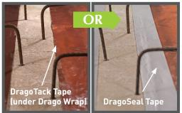
Onto Interior Grade Beams at Impediments: Seal Drago Wrap to concrete with **DragoTack Tape or DragoSeal Tape**.
