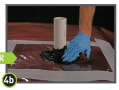
Seal around the base of the pipe with Drago Mastic. Note: apply using disposable glove, paint brush, or similar.
